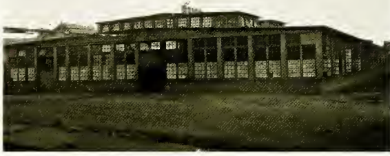
Addition to Sheldon Axle Co. Plant Conyngham Avenue
